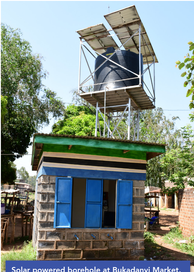
Solar powered borehole at Bukadanyi Market.
