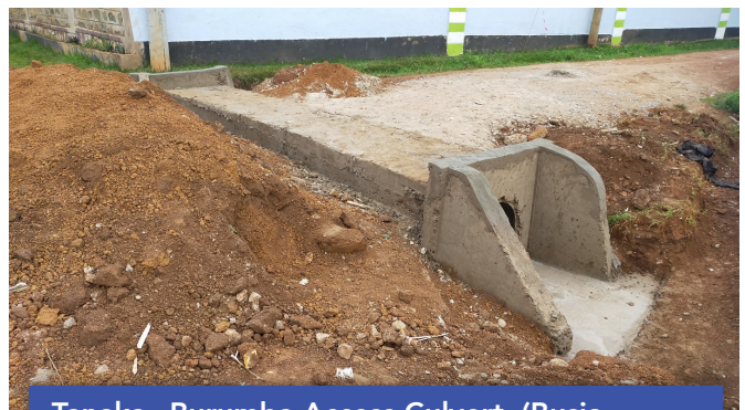
Tanaka -Burumba Access Culvert (Busia Municipality)
