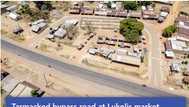
Tarmacked bypass road at Lukolis market.
