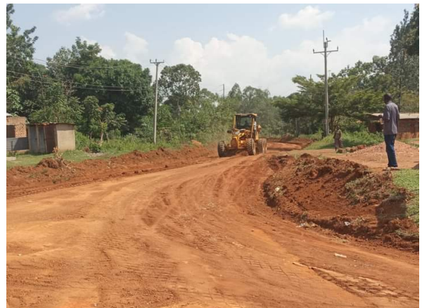
Muruka –Mung’abo – Kanyumba Routine Maintenance And Spot Improvement (Butula Sub – County)
